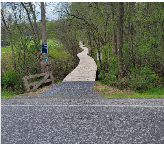
Figure 5: A New boardwalk Trail access from Ferry Road
