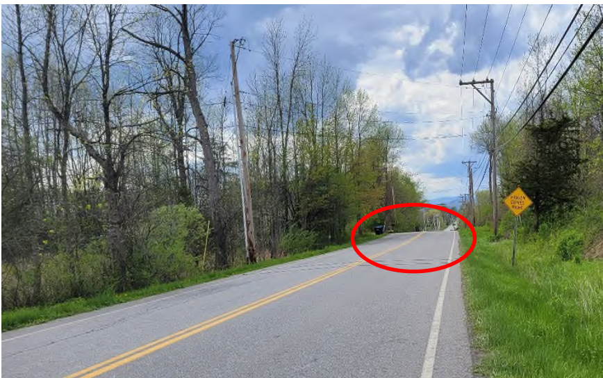
Figure 3: Difference in vertical elevation creating a crest, looking towards west
