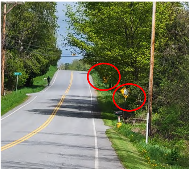
Figure 6: Vegetation obstructing signs, looking east
