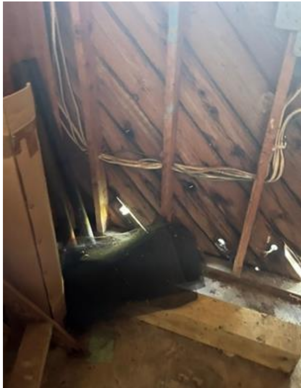
CONDITION OF SIDING
