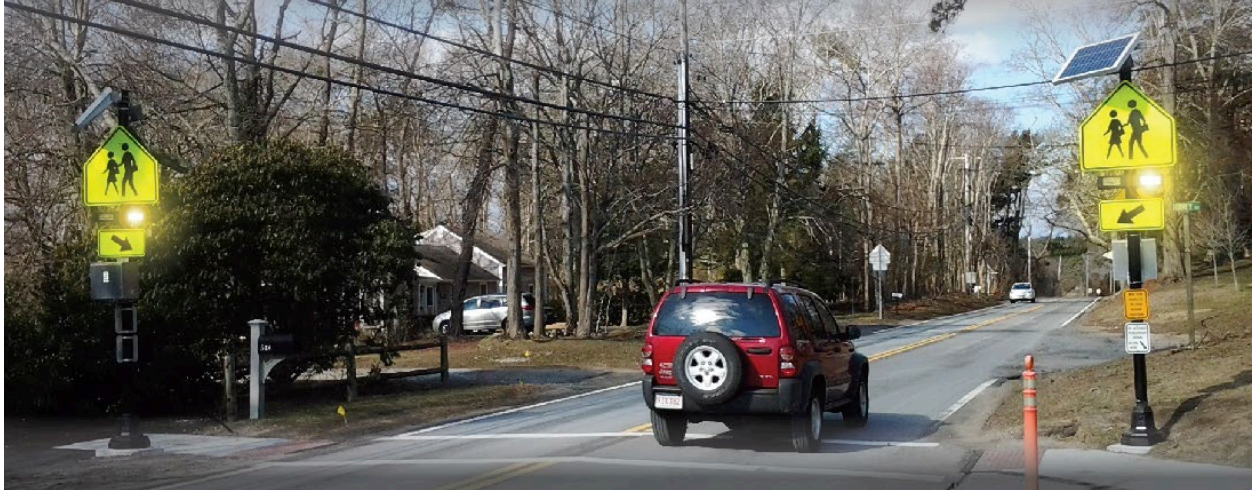
Figure 1 - Gate-posted RRFB installation at a school crosswalk
