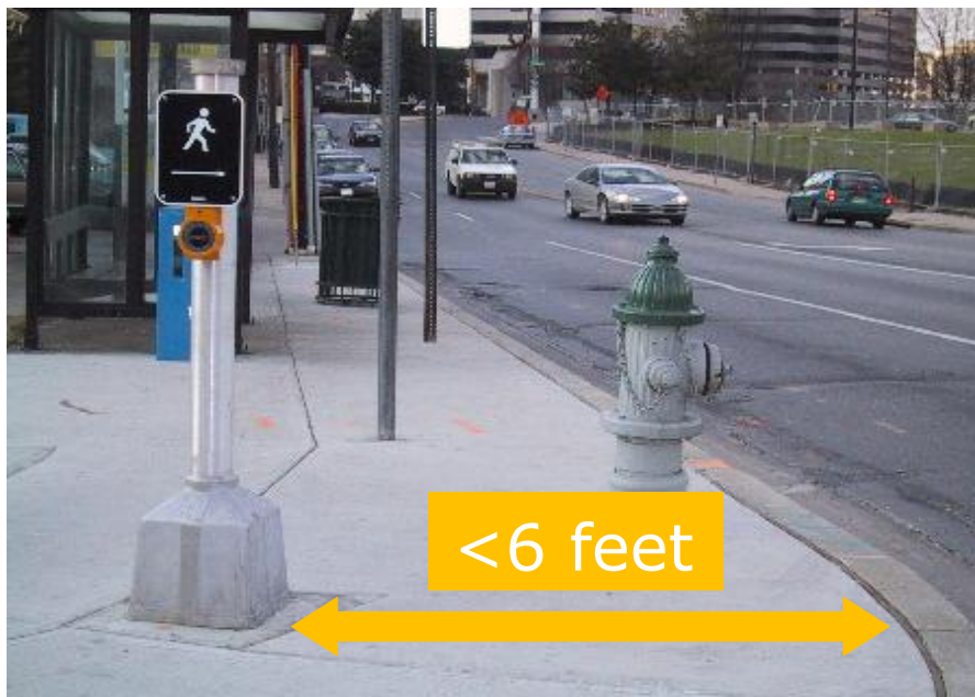
Figure 7 – Pushbutton relative to curb face
