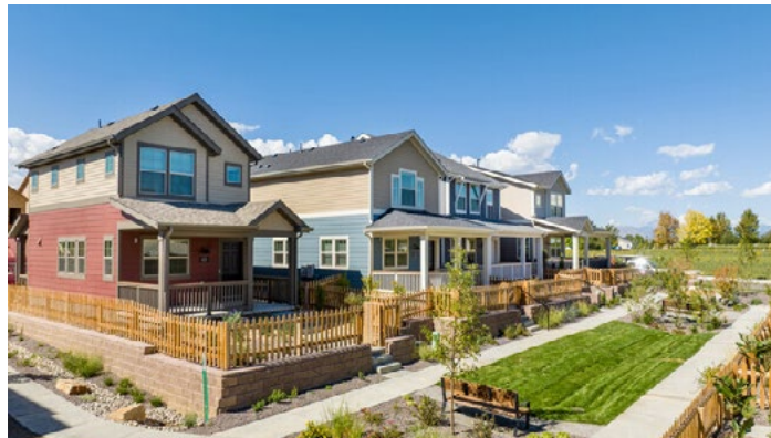
Single family homes on small lots with common space. Source: Cottages at Erie Commons
